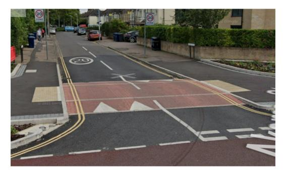
The crossing between points G and F on the attached plan will be similar to the photograph below. The road is raised and continues as a shared surface beyond the crossing point which again is raised to slow down vehicles and provide a level crossing for pedestrians. The footway continues for approx. 2m beyond the top of the ramp to provide a safe crossing for pedestrians.
